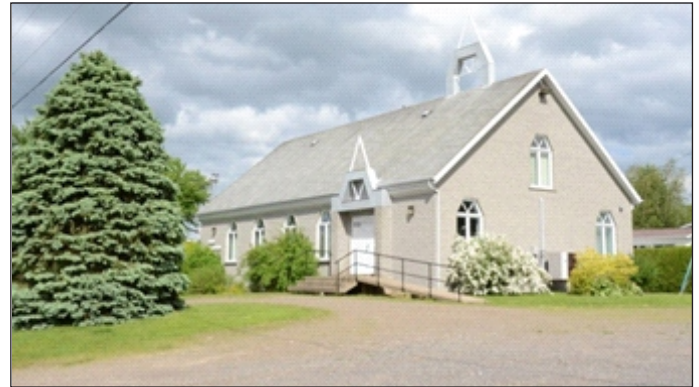
Fully paid for and renovated church building
